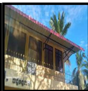
Repairing the Kottaramulla Public Library Nattandiya Pradeshiya Sabha – North Western Province Expenditure - Rs. 290,879.15
