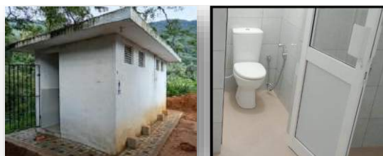
Providing public toilet facilities in Habarana Kekirawa Pradeshiya Sabha – North Central Province
