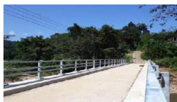
Construction of Bridge No. 5013+5014, Rathhota Narangolla Bridge, Matale
