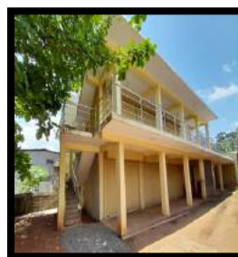
Construction of the Ukuwela Market Ukuwela Pradeshiya Sabha – Central Province Expenditure - Rs. 10,656,763.54
