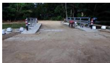
Construction of Bridge No. 5028, Hambantota Angunakolapalassa Jadura Bridge
